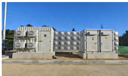
China Huaneng Group, Power Construction Corporation of China and other distributed Photovoltaic 10kV direct hanging outdoor air-cooled SVG projects
