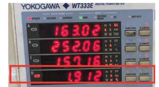
After mitigation, the current harmonic distortion rate was 1.9%.
