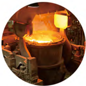
Heating Furnace Equipment
