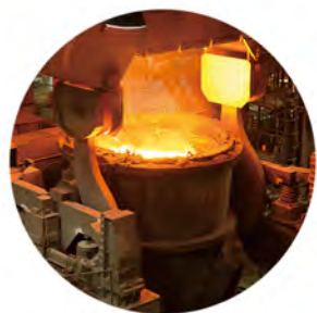
Heating Furnace Equipment
